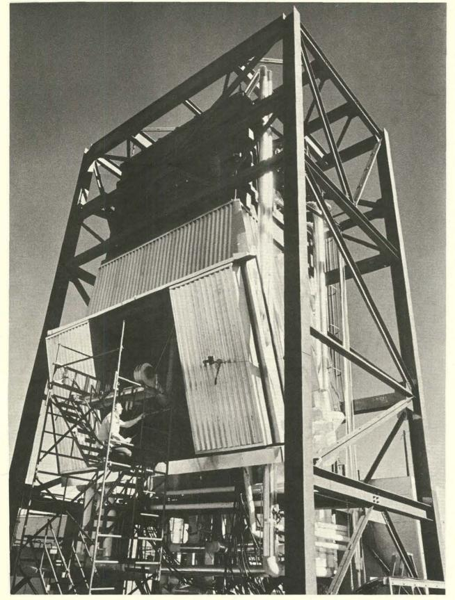
SOLAR RECEIVER STRUCTURE, possibly destined for top of the "Power Tower" in Area III, is undergoing test at the Radiant Heat Facility. Phil Class (9331) is near area between doors where concentrated beams of 200 mirrors tracking the sun will be focused. Receiver wall is now lined with 2000 infrared lamps which simulate the five megawatts thermal energy the receiver will sustain during operation.
